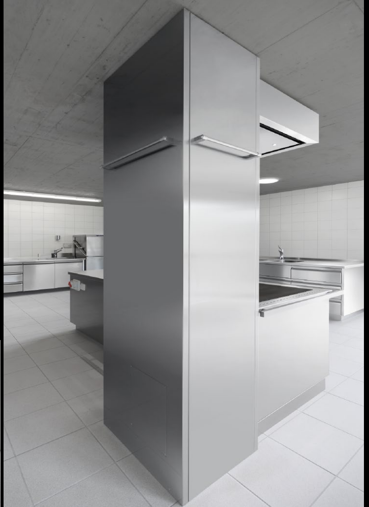
Column completely clad in stainless steel
