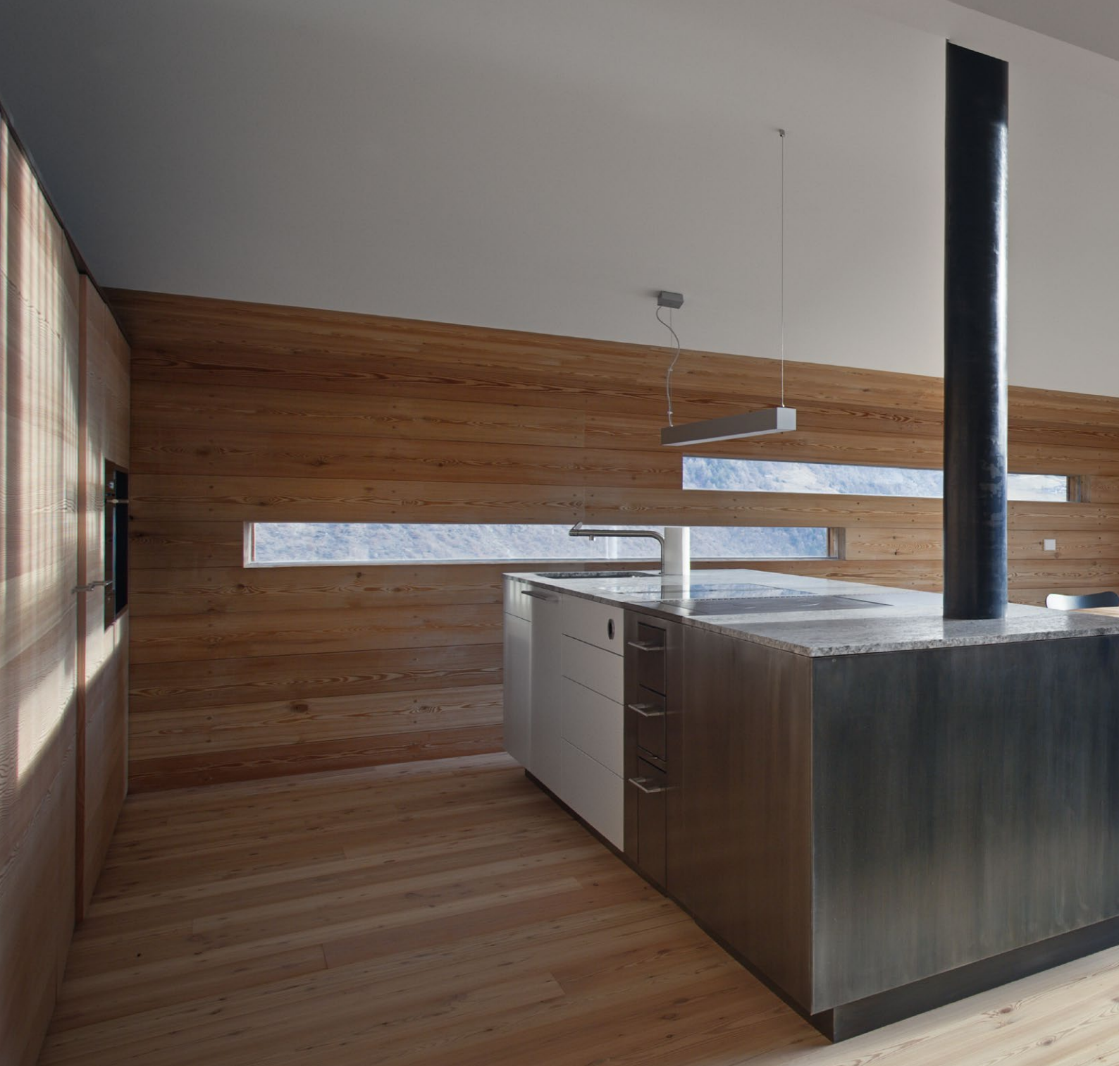
Special kitchen stove with perimeter flue gas that allows heating the entire living area
