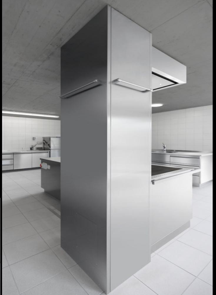
Column completely clad in stainless steel
